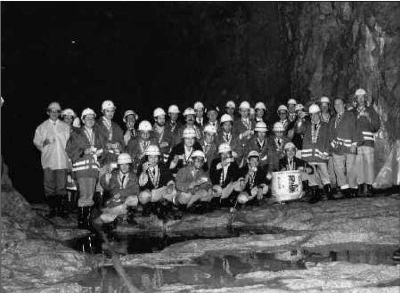
Tunnelling in Hong Kong for the Mass Transit Railway.
